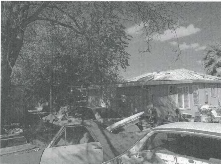
Photo 10: Looking northwest at the residential home
