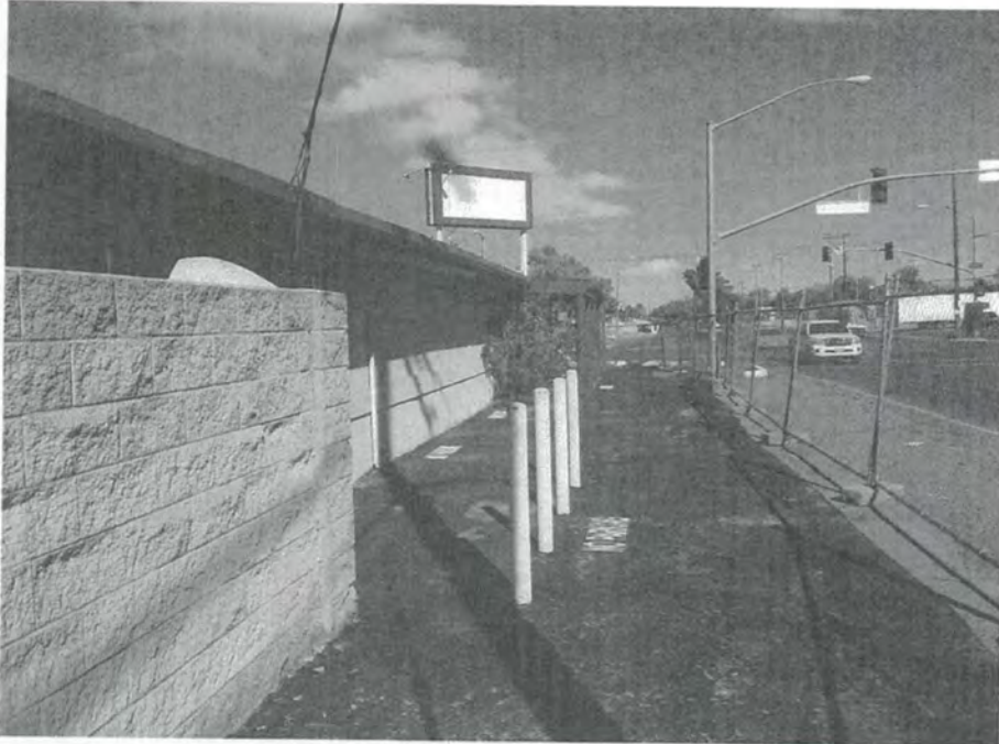
Photo 12: Looking north at the side of the building
