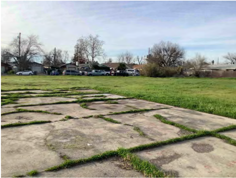
Photo 1. Concrete slabs, facing SW, January 21, 2022.
