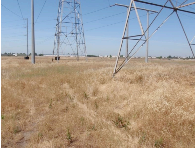
Photograph 2. View of top of north pedestal, looking southwest (5/22/09).
