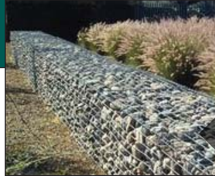
Low Gabion Wall
