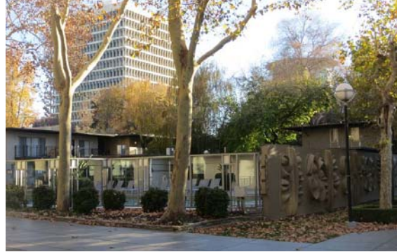
Jacques Overhoff's concrete relief wall
