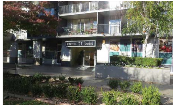
Existing Capitol Towers multifamily complex
