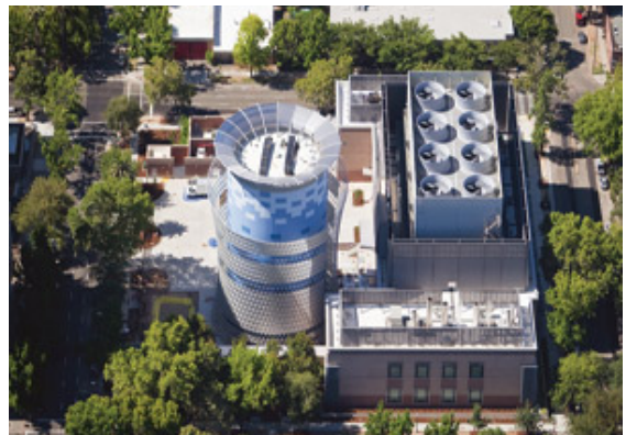
Neighboring State Central Utility Plant
