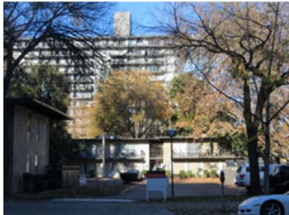
① View to Site from P Street
