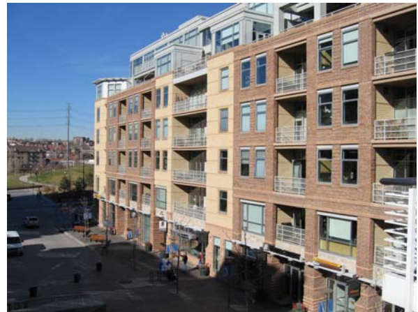
Materials shall vary in tandem with massing to differentiate uses or tenants.
