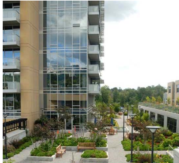
Towers should appear transparent by maximizing the use of glass, curtain wall systems, and balcony railings.
