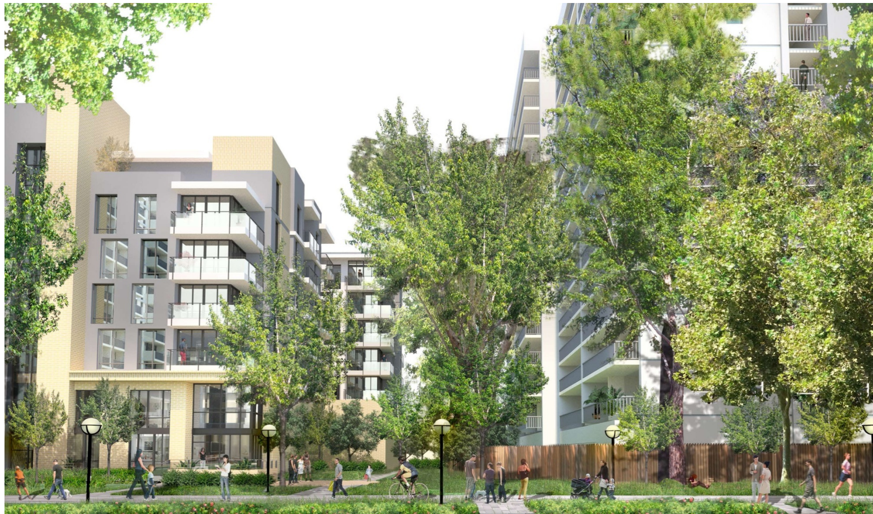
Figure 2.11 Conceptual View of Streetscape at N Street Entrance to the North-South Promenade
