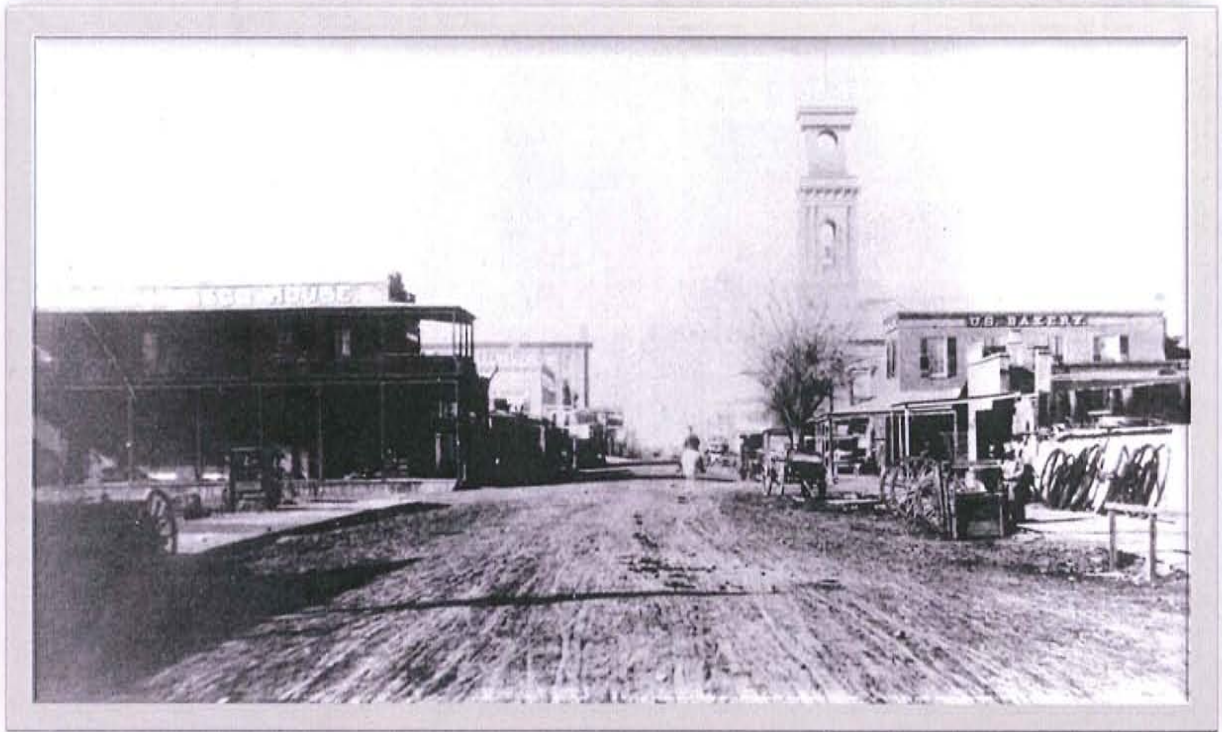
This photograph shows the 700 block of K Street, ca 1865. The tower of St. Rose of Lima cathedral is on the right, at the corner of 7 th and K.
