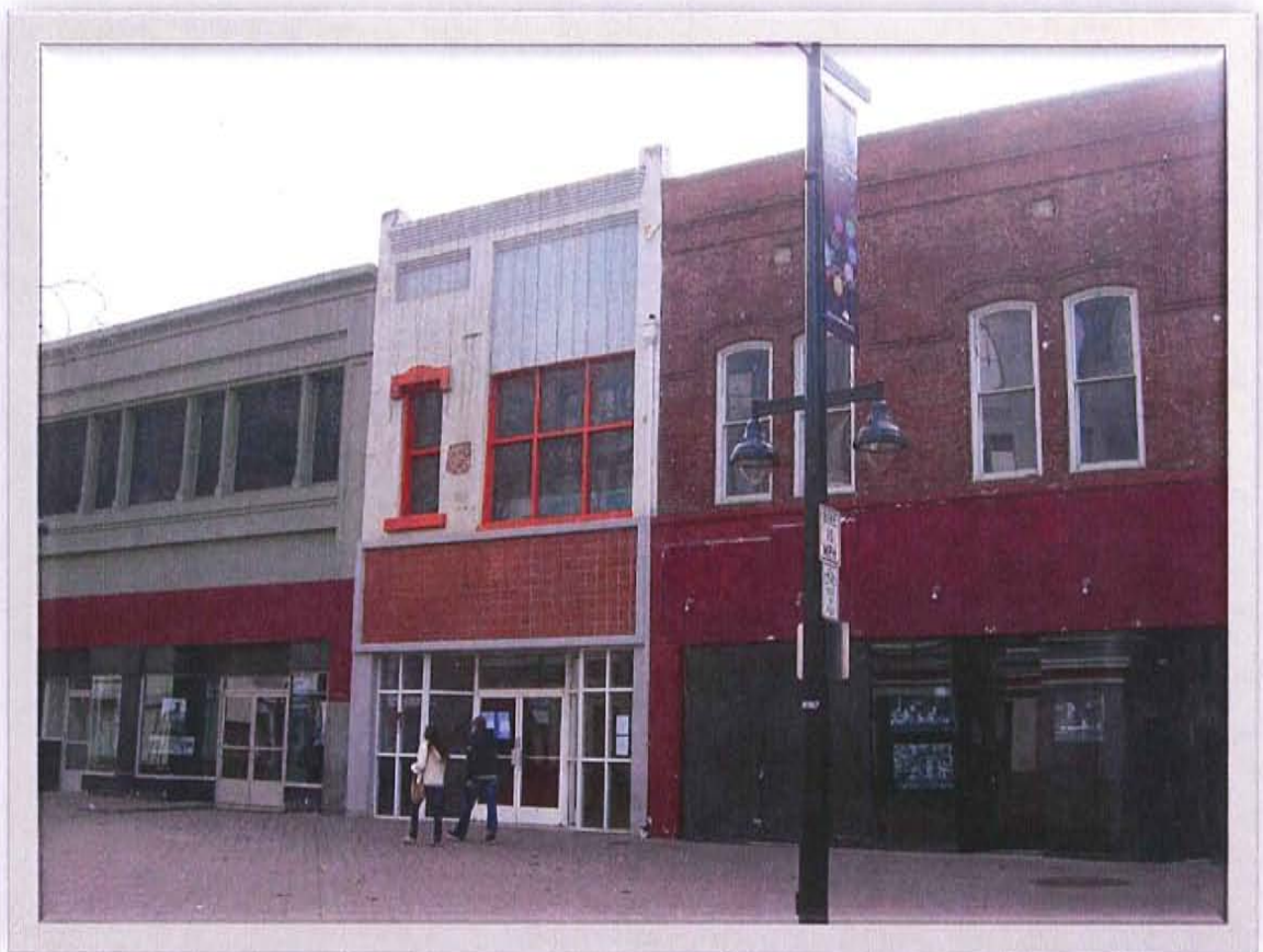
716 K Street – View to the south.
