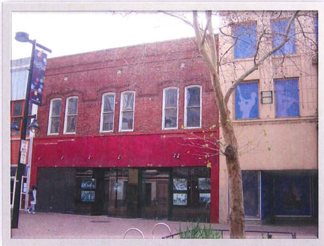
712, 714 K Street – View to the south.
