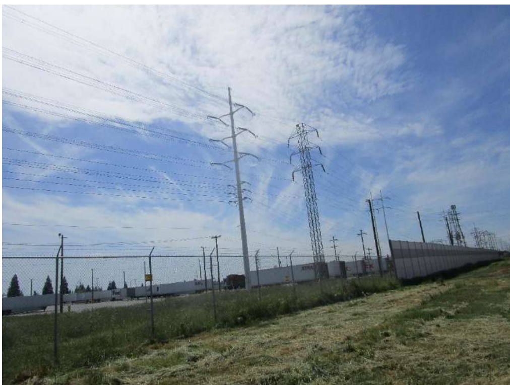
Photo 20: View of adjoining property to the south and high-voltage power lines.
