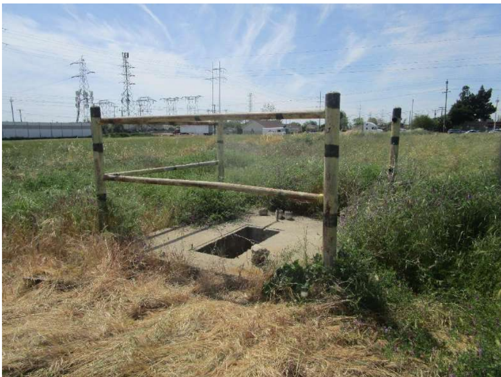
Photo 12: View of concrete vault in center of subject property.
