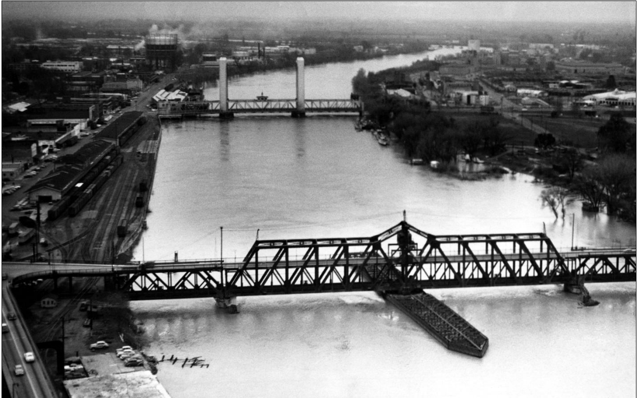
Figure 28. The I Street (foreground) and Tower (background) Bridges pictured in December 1955. [Center for Sacramento History, Frank Christy Collection, 1998/722/0272].
