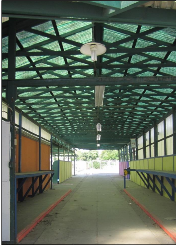
Photograph 4. Overview of a west hallway (view to west)
