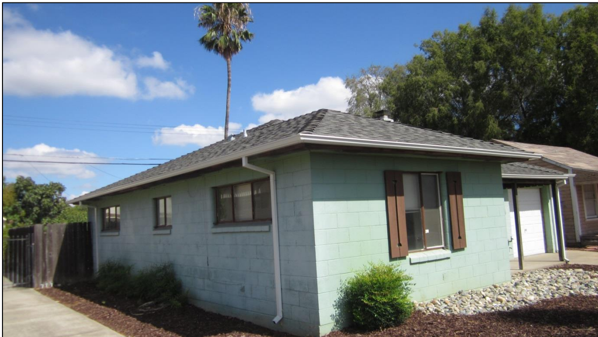
Photograph 8. Overview of West Elevation (view to northeast)
