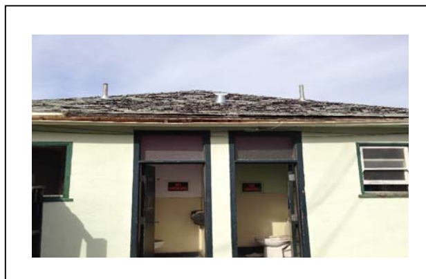
Photo 5: Abandoned buildings with potential for roosting bats.
