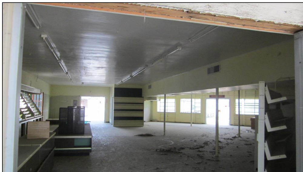
Photograph 5. Partial view of the 1962 Office Addition (view to southwest)
