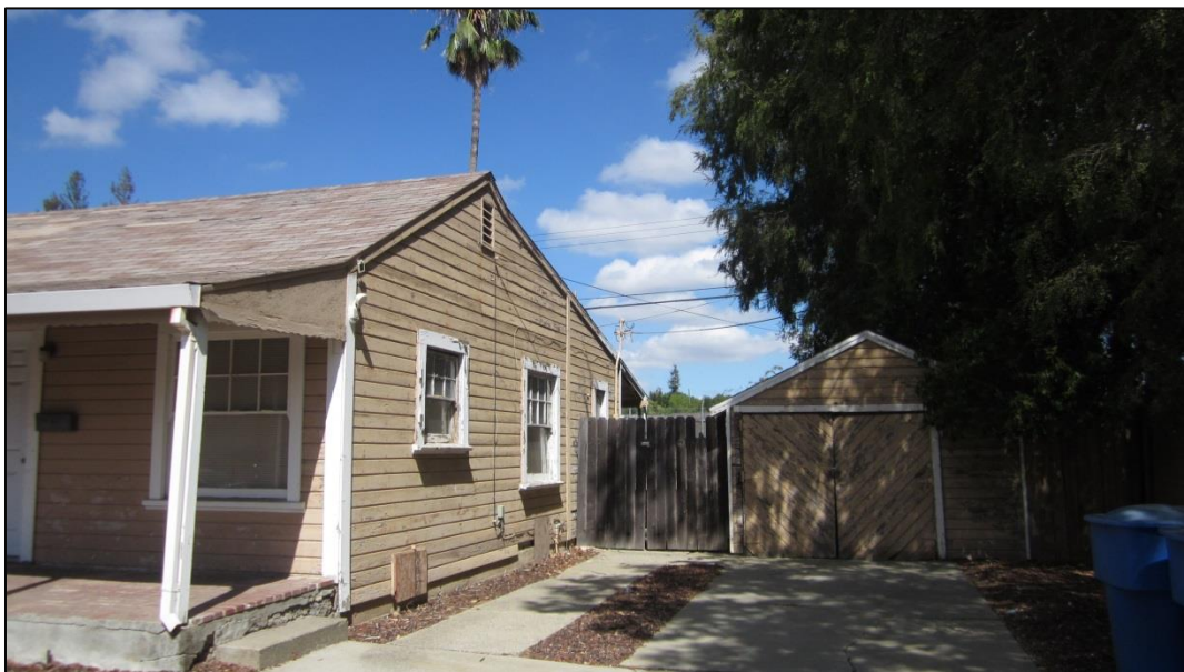
Photograph 11. Overview of East Elevation (view to northwest)
