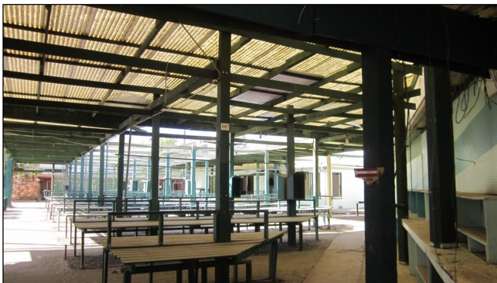
Photograph 3. Overview of a south hallway (view to south)
