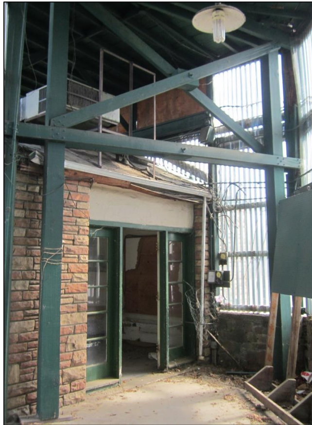
Photograph 2. Partial view of the garden shop (view to northeast)
