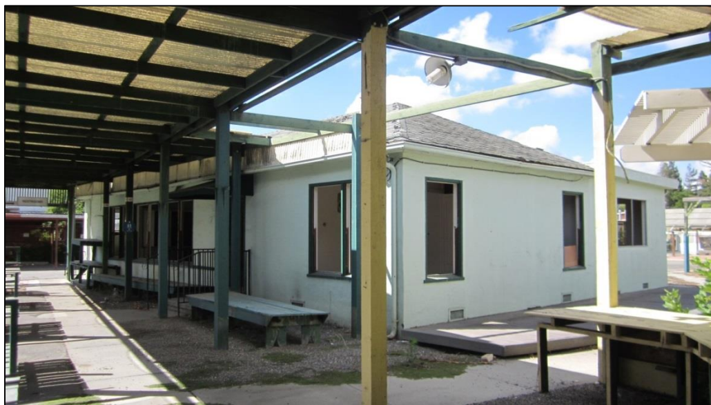
Photograph 7. Overview of Restroom Building (view to southwest)
