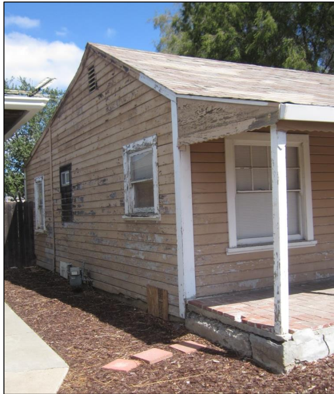
Photograph 10. Overview of West Elevation (view to northeast)
