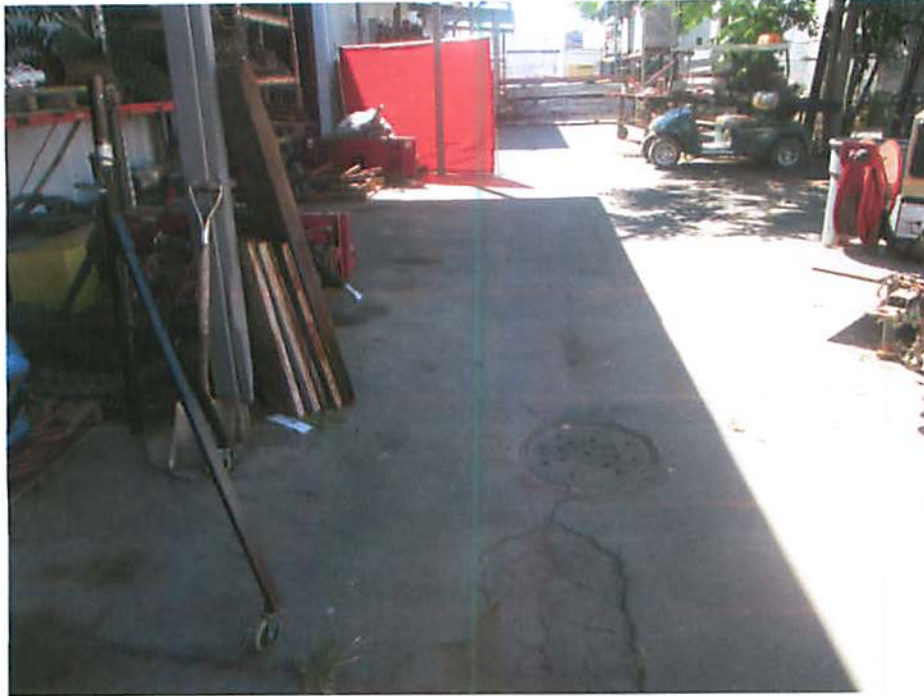
Photo 9: Looking at the storm drain inside the property
