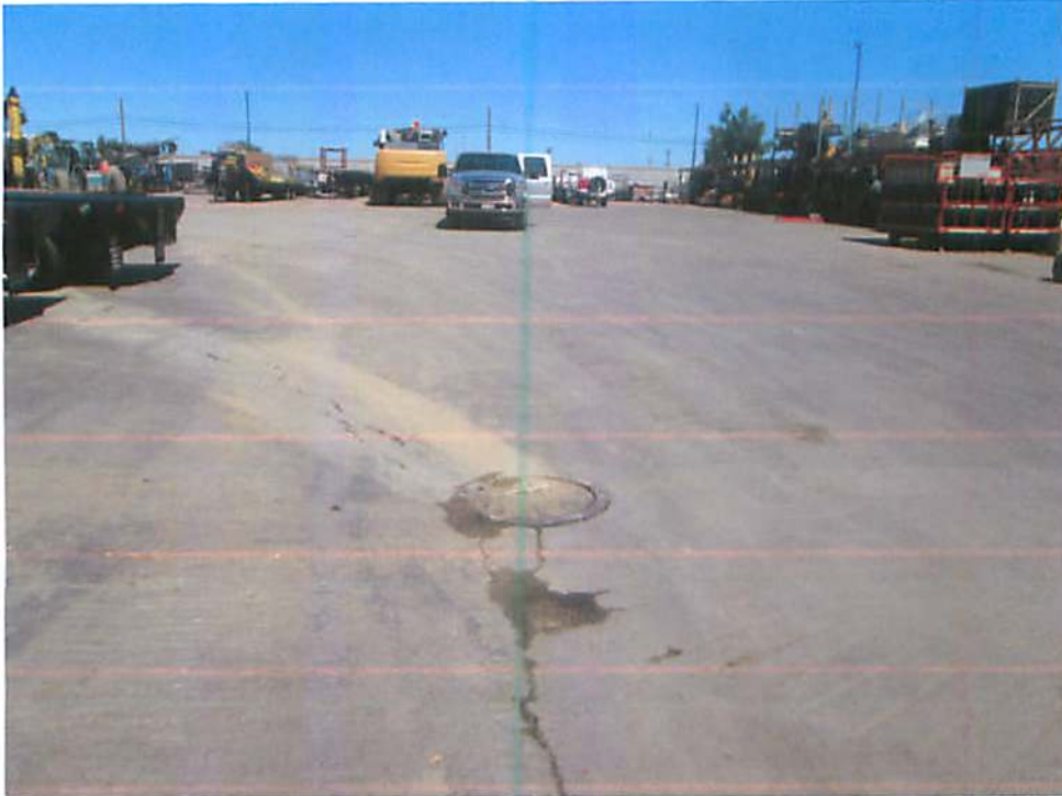
Photo 17: Looking at another storm drain in the yard area
