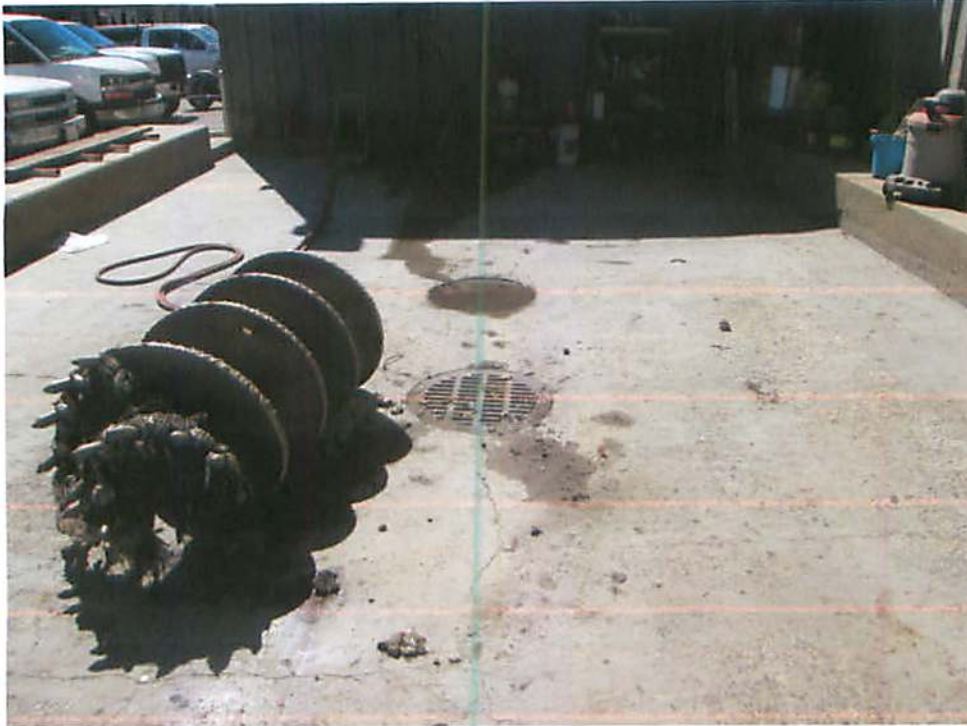
Photo 15: Looking inside the wash area
