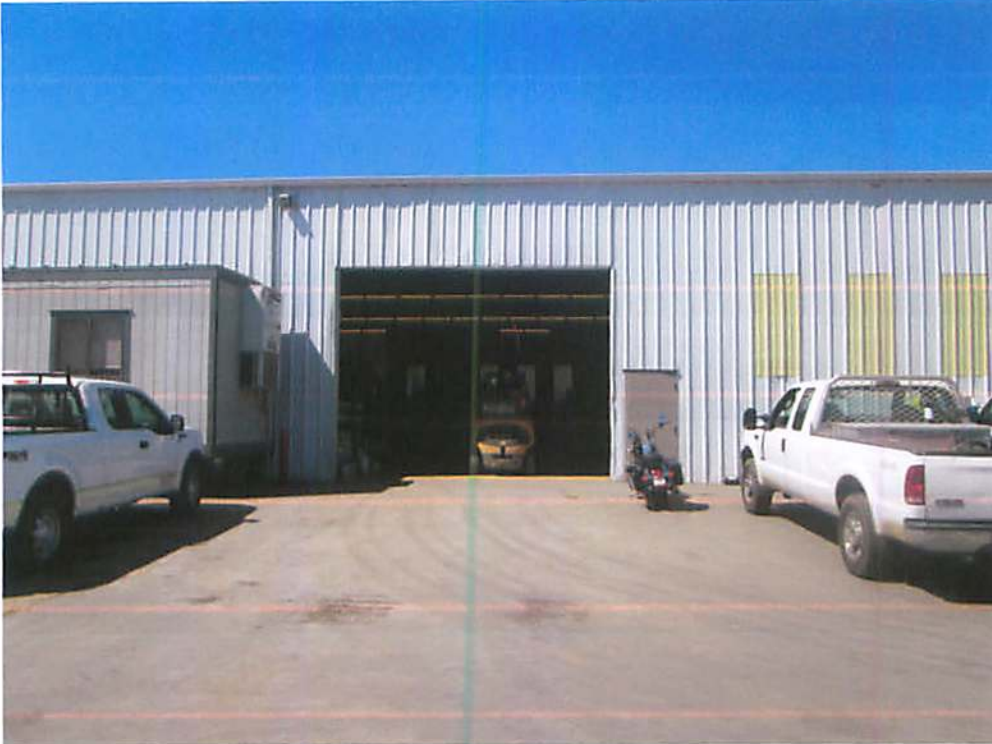
Photo 19: Looking south at the metal warehouse building
