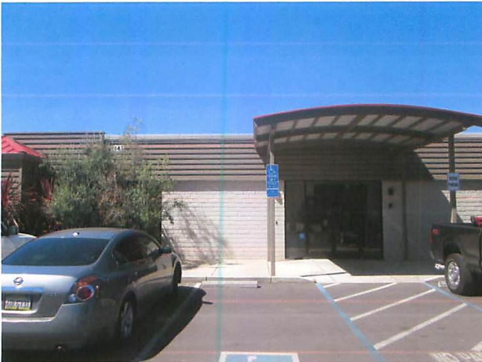
Photo 20: Looking south at the entrance to the office area
