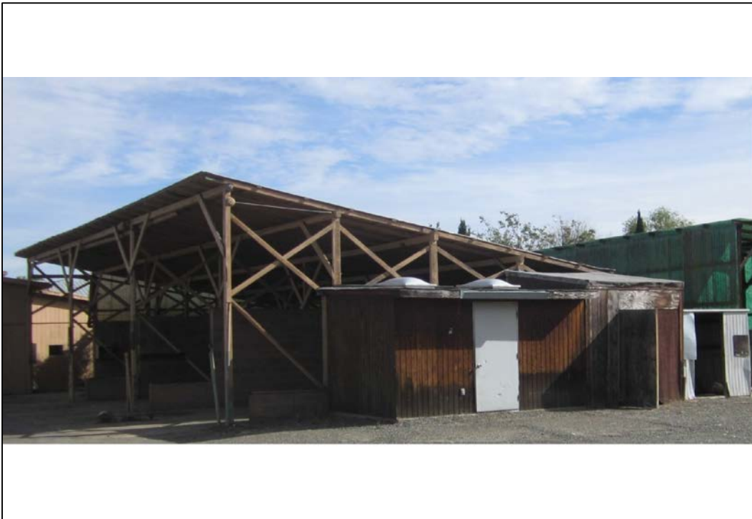
Figure 4.1-3 Viewpoint #2 - On-Site Storage Shed
