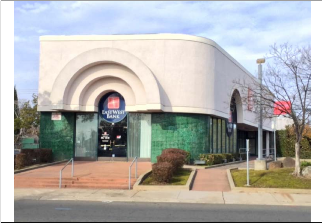
Figure 4.1-11 Viewpoint #9 - View looking west from Freeport Boulevard of East-West Bank
