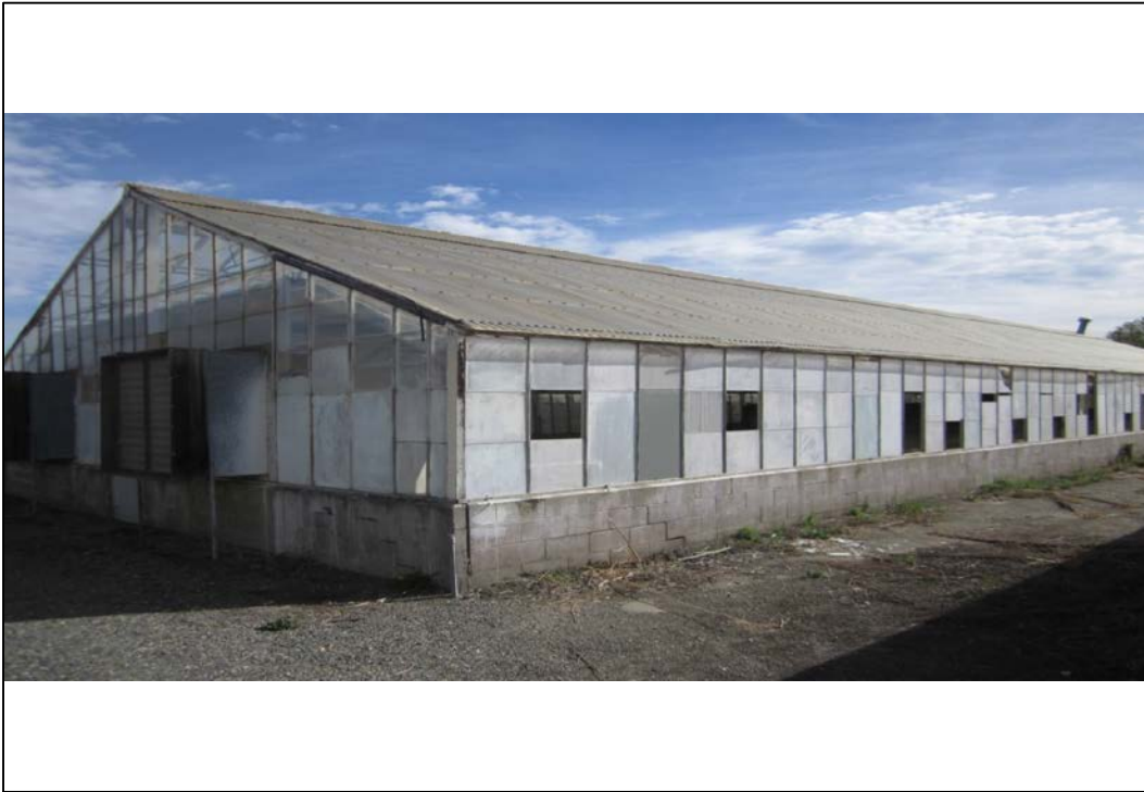
Figure 4.1-2 Viewpoint #1 - On-Site Greenhouse
