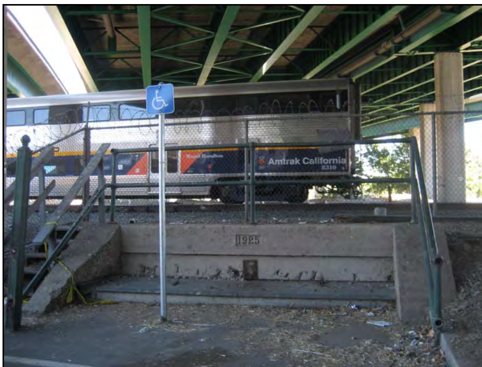
Southern Pacific Tunnel/Pedestrian Subway, south portal. View north. July 2008.
