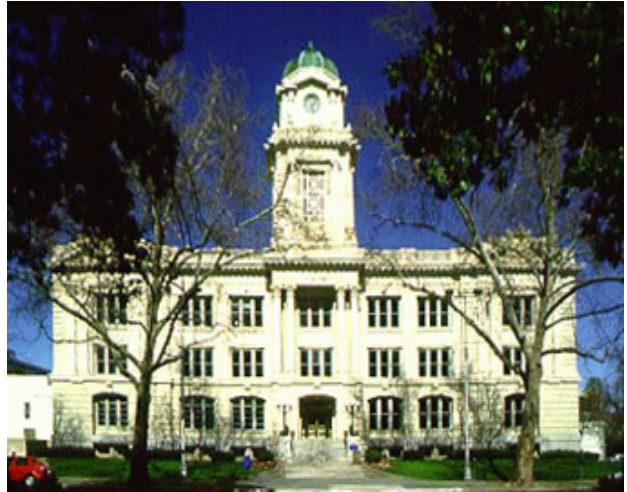
Sacramento's City Hall at 915 I St.
