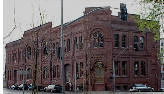
Station A at 6 th and H St.
