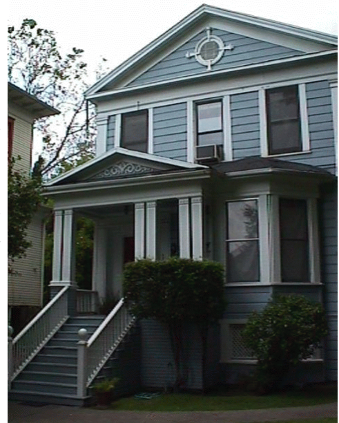
Hartley House at 1107 F St.
