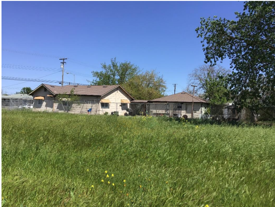
132 Silver Eagle Road, west and south facades. April 13, 2023, IMG_1904
