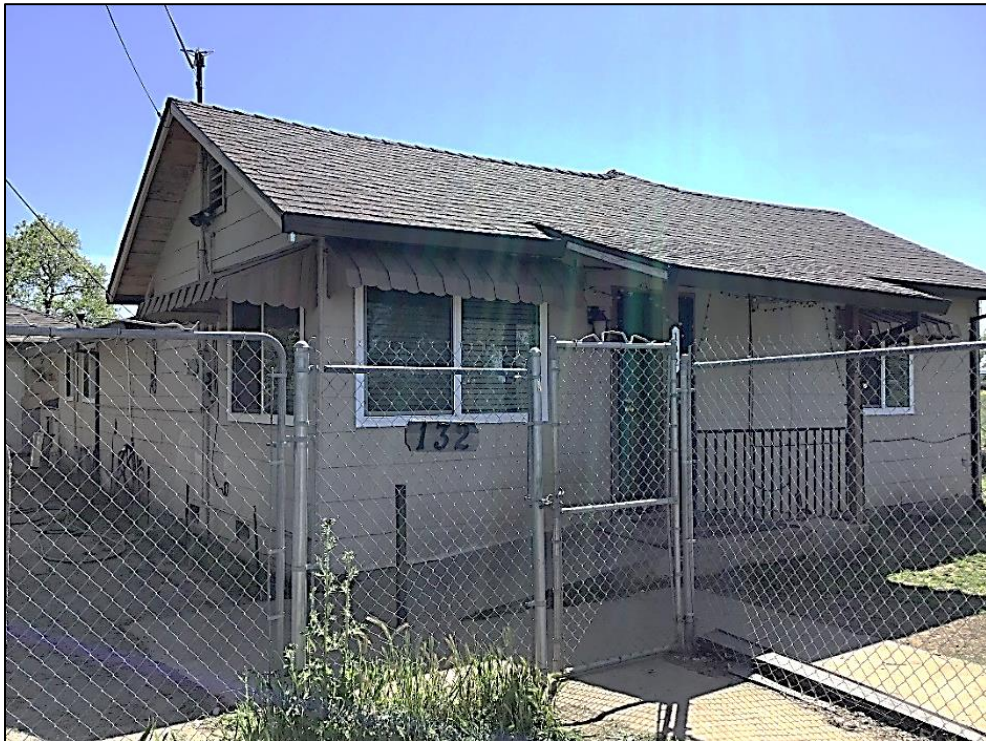
Figure 8. 132 Silver Eagle Road, north and east facades. April 13, 2023
