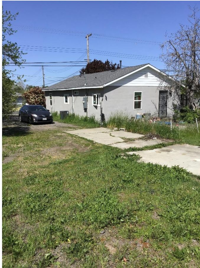
150 Silver Eagle Road, west and south facades. April 13, 2023, IMG_1935
