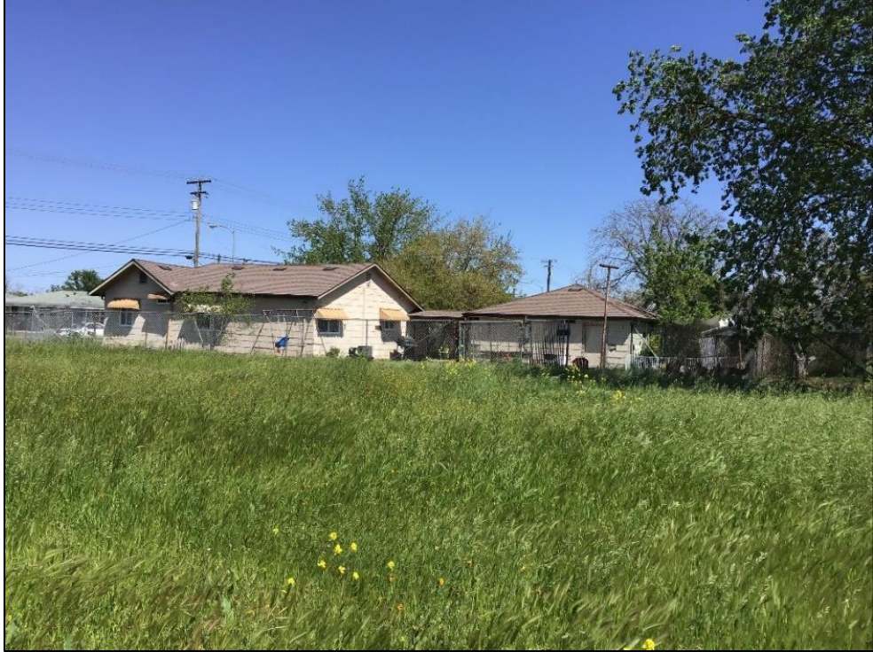
Figure 7. 132 Silver Eagle Road, west and south facades. April 13, 2023
