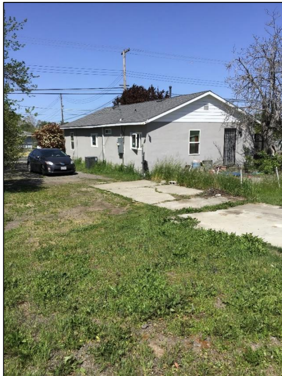
Figure 10. 150 Silver Eagle Road, west and south facades. April 13, 2023
