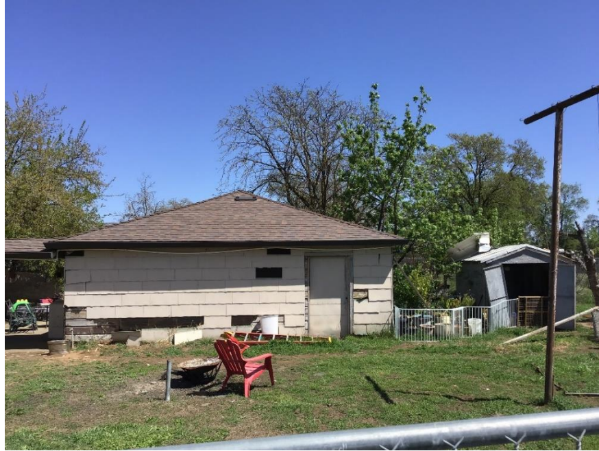
132 Silver Eagle Road, west façade of garage and shed, view east. April 13, 2023 IMG_1916
