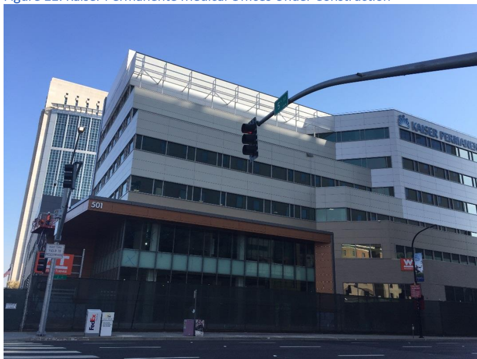
Figure 11: Kaiser Permanente Medical Offices Under Construction
