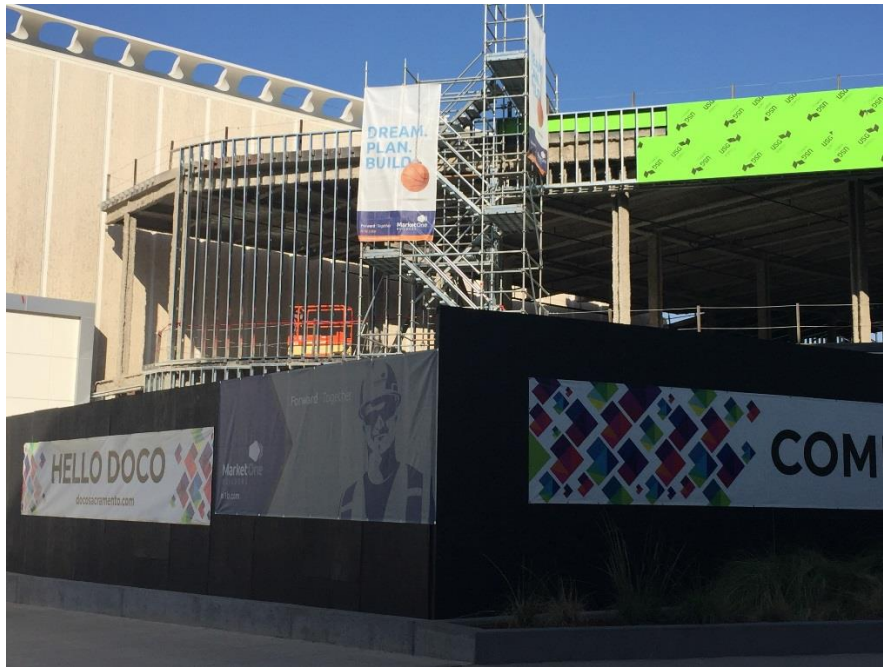
Figure 10: Construction of the Downtown Commons Area Near Macy's
