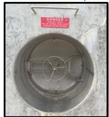
Figure 25: Example Entry Point for a Confined Space
