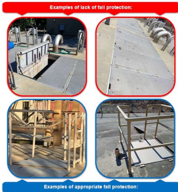
Figure 27: Examples of Haphazard Fall Protection
