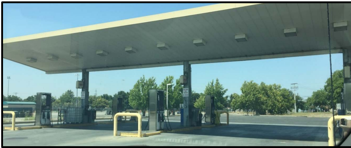
Figure 20: Meadowview Facility Fueling Island
