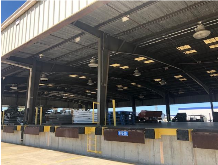
Figure 9: Part of Dock at the City’s North Area Corporation Yard
